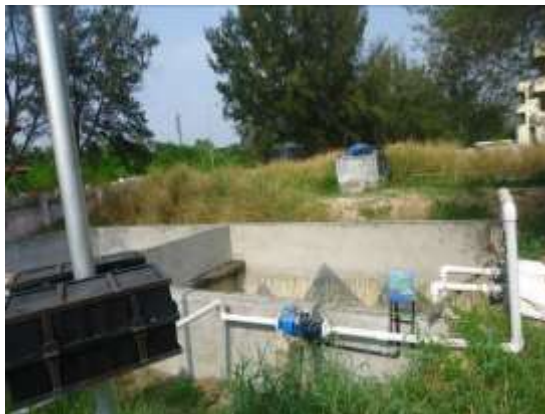
Renovation of Primary collection tank
